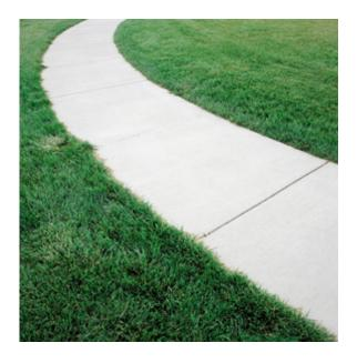
2. The walkway consists of a 4-inch deep layer of gravel and then a 4-inch deep layer of concrete. Based on the dimensions of your design, you will need to decide how much gravel and how much concrete will need to be delivered in order to make your walkway. Gravel and concrete are both measured in cubic yards.
